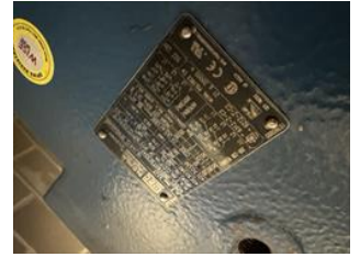
Ah1 return motor. Motor bearings are 6312zc3 and 6212zc3
