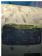
6 supply fan 2 motor bearings are 6311 and 6312
