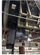
9 return. Cannot access fan bearings
