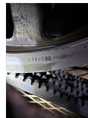
Ah11 supply air handler pulley 2 3/8" shaft. Pulley number is 5B5V160
