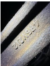
4 groove 8 supply fan pulley. 4R5V212
