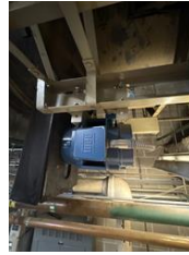
Ah1 return motor cannot access fan bearings
