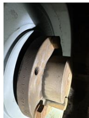
Ah10 supply motor shaft 2 1/8"
