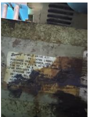
6 supply fan 2 Cannot identify pulleys or belts on tag
