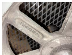
Ah11 return air handler pulley
