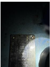
Ah11 supply. Motor bearings are 6316c3 and 6314c3
