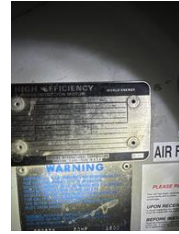
7 return fan 2. Motor bearings are 6310zc3 and 6310c3
