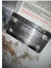
8 return motor1. Motor bearings are 6310zc3 and 6310
