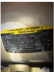
8 supply motor 1. Motor bearings are 6312 and 6313
