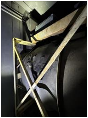
Ah5 cannot access fan bearings Ah5 m1
