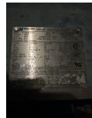
7 supply motor 1 identical to 8. Motor bearings are 6314 and 6311
