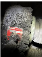
Ah11 return inboard. Bearing is SPB1000NEx with a 2 7/16" shaft
