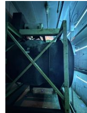
6 supply motor 1 cannot access fan bearings
