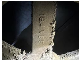
9 supply fan pulley 2 15/16 shaft. 18.4xB5
