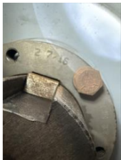
Ah10 supply fan shaft. 2 7/16"
