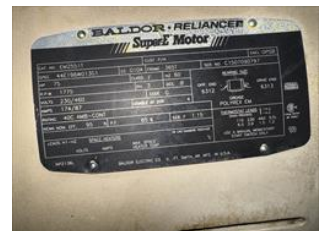
7 supply motor 2. Motor bearings are 6312 and 6313
