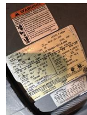
8 supply motor 2. Motor bearings are 6313 2Z JC3 and 6212 2Z JC3
