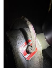
Ah11 return output air handler. Output bearing is SPB1000EX with a shaft size of 2 7/16"
