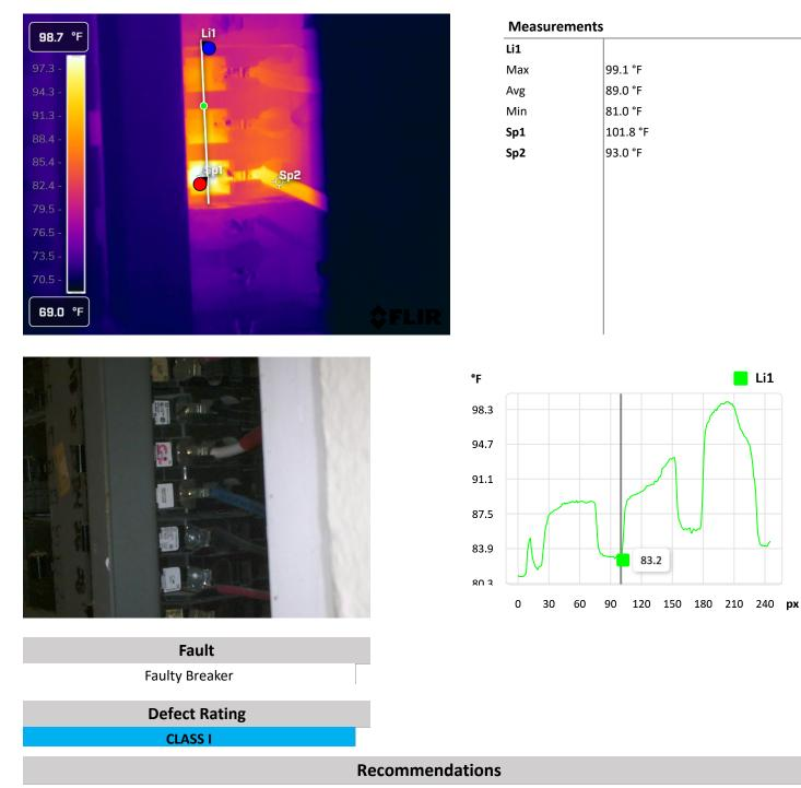
Breaker has internal heat with minimal load. Breaker likely has internal issue and should be replaced as time allows.
