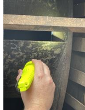
East fan is rubbing the shroud, it'll have to be done later
