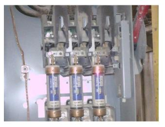
Fault Loose worn fuse clip Defect Rating CLASS II
