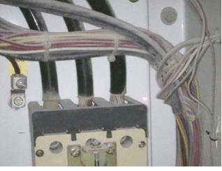
Fault Connection issue Defect Rating CLASS I
