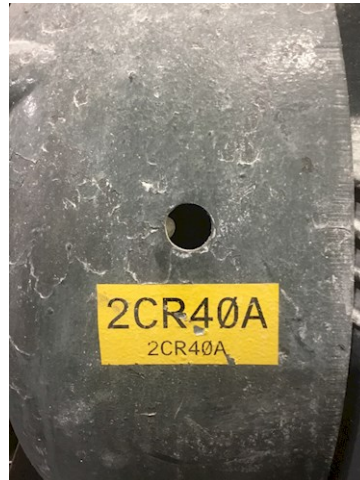
ODE grease fitting not lined up.
